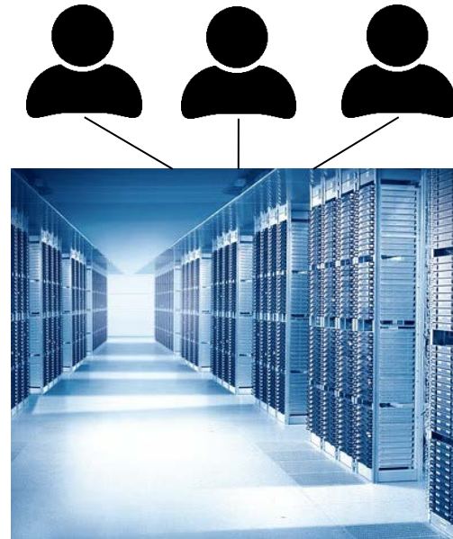
Strato Data Centre, cloud ^
